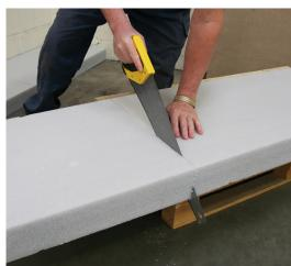
**5** Cut both parts of the Plinth to size by cutting along the pencil lines.
