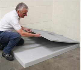
**2** Sit the Showerlay on top of the Plinth making sure the Showerlay is not over hanging the Plinth on any sides.
