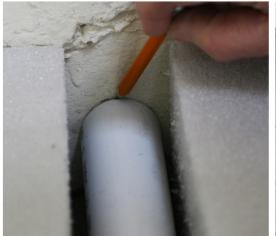
**7** Lay the Plinth into position then mark the wall for the pipework. Now once again remove the Plinth and drill out the hole drawn on the wall.
