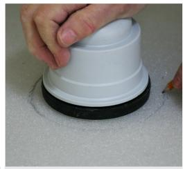
4 Remove the Showerlay and place the Dallmer drain upside down over the circle drawn on the Plinth. Now draw a pencil line around the Dallme drain leaving roughly a 10mm gap.
