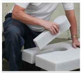
**6** Cut out the hole for the drain and also space for the pipework.
