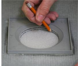
**3** Mark out the position of the hole and also draw around the edges of the Showerlay with a pencil onto the Plinth.
