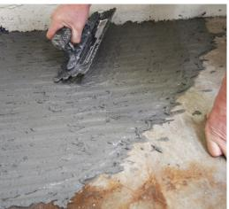
8 Now fix down the Plinth to the floor using a full bed of flexible cement based tile adhesive. Use the adhesive to help level any uneven floors.
